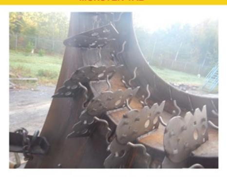
To prevent flow bypassing, as I mentioned previously, Shell uses what is called a vapor stop. You can see there that it is a ring of steel that goes around the vessel and protrudes into the refractory.
