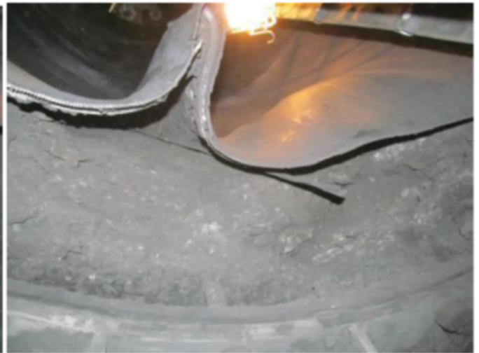
Picture-2(b): Last panel of outside reactor grid found fully bulged with huge coke build up
