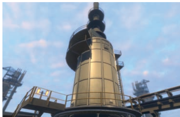
The VR simulation trains employees by using three different modules to familiarize them with the hazards of lighting a fired heater and build their competency.
